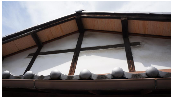
Typical wooden framework for the Shake-machi district
